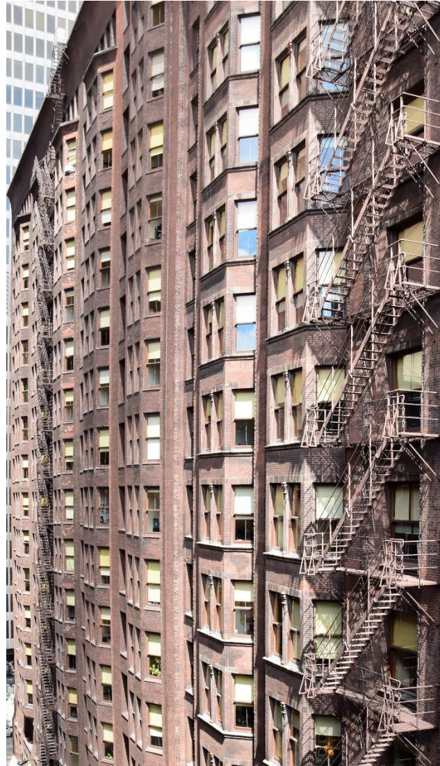
Monadnock Building Burnham & Root, 1891; 16 stories. World's tallest loadbearing brick building. Walls are 6' thick at the base.
