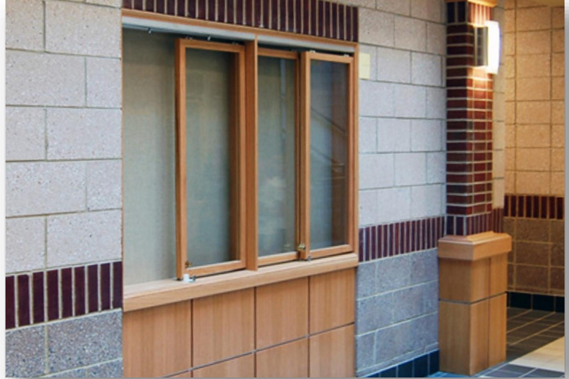
CMU interior finish
