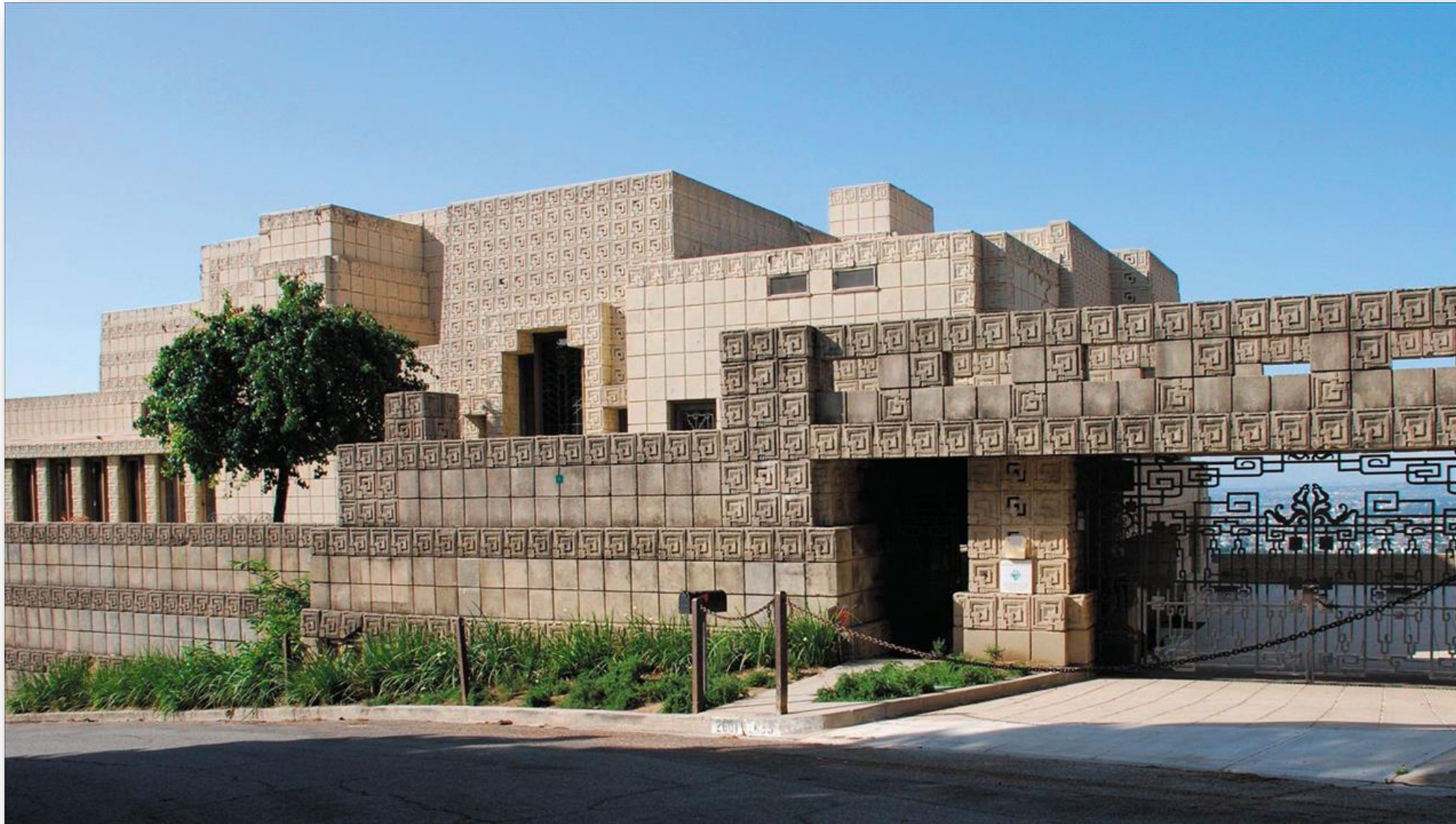
Ennis House, Los Angeles, Frank Lloyd Wright, 1924
