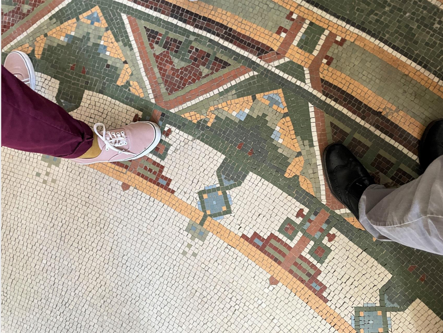
Sullivan Center (Carson Pirie Scott), Chicago
