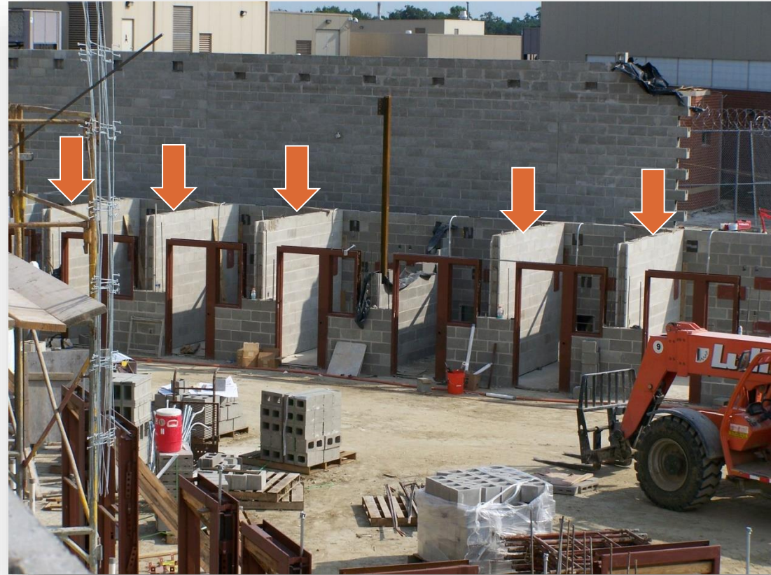
Walls set in place by crane
