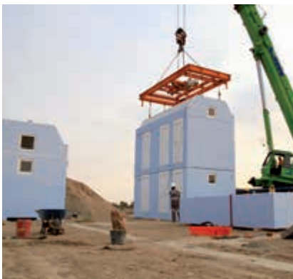
Top: Modular housing project. The room modules were produced using three modular moulds, roof and stair moulds and a battery.
