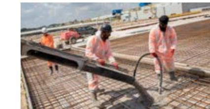
This trial demonstrated the potential to use very high ground slag (GGBS) contents in excess of 90 per cent, as an alkali activated cementitious material conforming to BS EN197, the standard for cementitious materials allowed to be used in ready mixed concrete, to significantly reduce carbon emissions, whilst still producing a quality finish and allowing normal construction and demoulding times.
