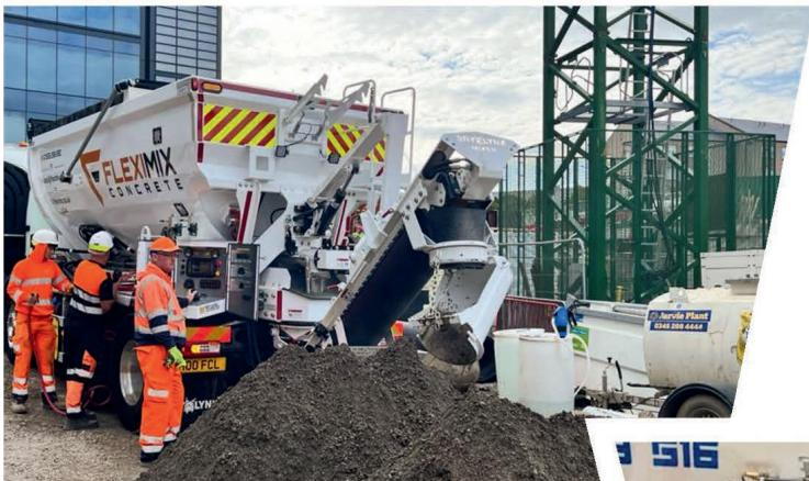
A volumetric mixer precisely proportions out cement, sand, stone and water on-site. No mixing as you drive, no getting stuck in traffic while the mix in the back hardens and changes properties.
