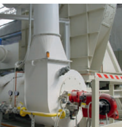
Type LF10 LOMA heater with a natural gas burner, 2008
