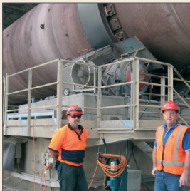
Mr. Phil Immes & Mr. Brad Lewis Golden Bay Cements Rotary Kiln with CJC® HDU 27/27 Mobil Fine Filter installed
