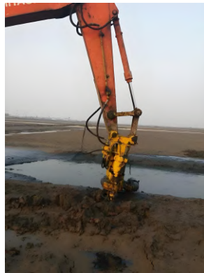
200THY75-6P+2 Expro-11 Installation on Hitachi Ex-200 for Sludge Handling. (New Zealand)
