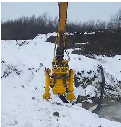
300THY110-6P + 2 Expro-15 on Sany 750 Excavatoe. (Russia)
