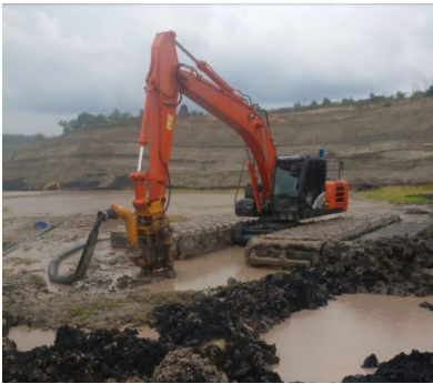
200THY90-6P + 2 Expro-11 Mounting on Komatsu 36 ton Excavater in Quarry. (UK)
