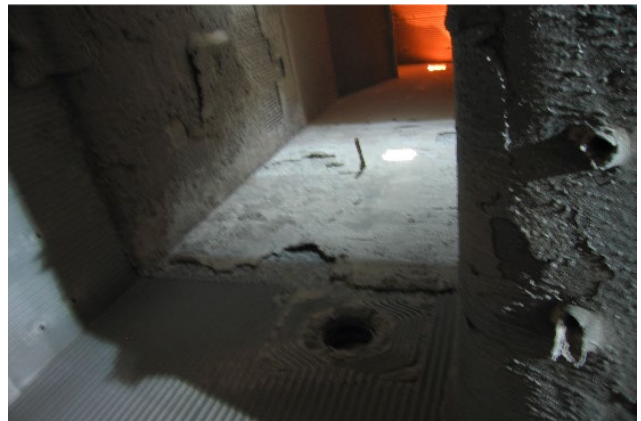
Almost New Refractory
