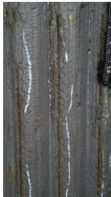
Field services – on site weld overlay
