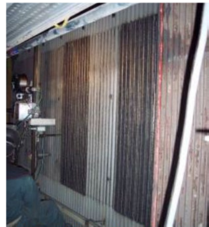
Field services – on site weld overlay
