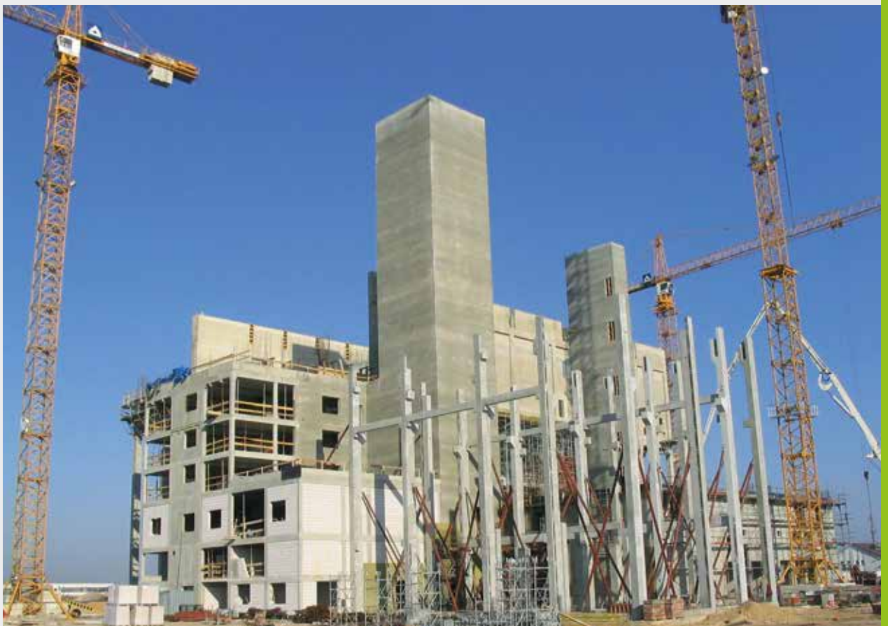
EfW plant under construction in Zorbau (Germany)
