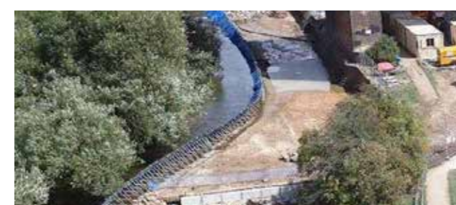
Coffer dams to unlimited length
