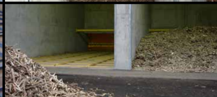
Hydraulic discharge device (pulling cylinders)
