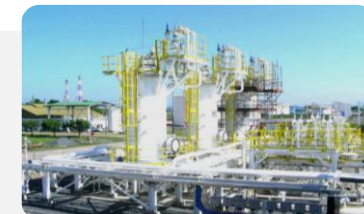
Condensate Mercury Removal System
