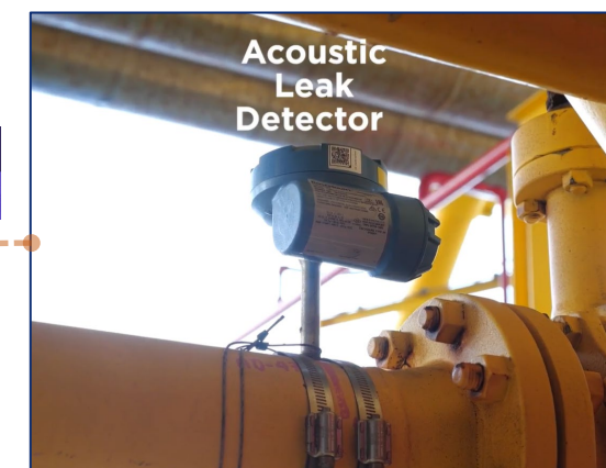
early detect PSVs and flare valves passing
