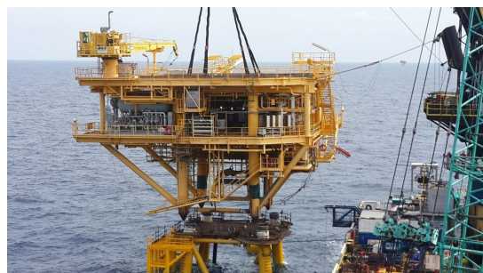
Wellhead Platform Topside Reuse
