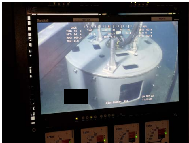
3. Cleaning using WHCT
