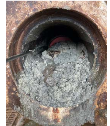
Pipeline pigging operation
