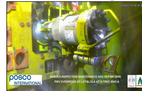
< LOT Installation on top of LOLA >
