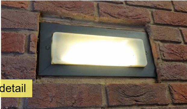
Example of original projecting rectangular diffuser light
