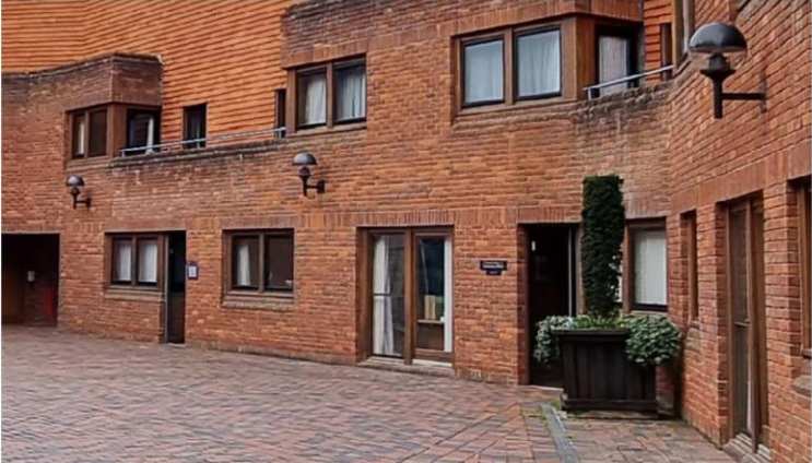
Non-original external globe lights which are similar in form to the originals
