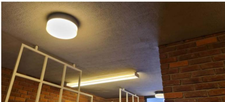
Circular light fittings which are likely to be original, with additional fluorescent tube lighting added
