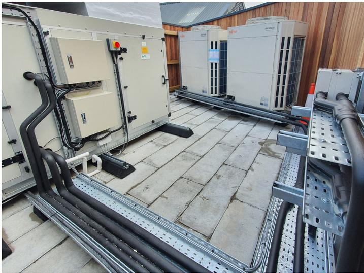
Fujitsu Airstage V-III providing direct expansion cooling and heating via AHU
