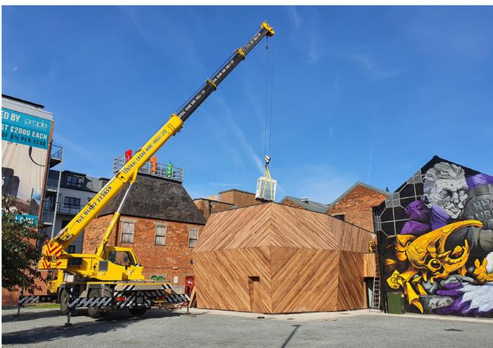
Fujitsu Airstage V-III heat pump VRF being positioned on the roof plant compound
