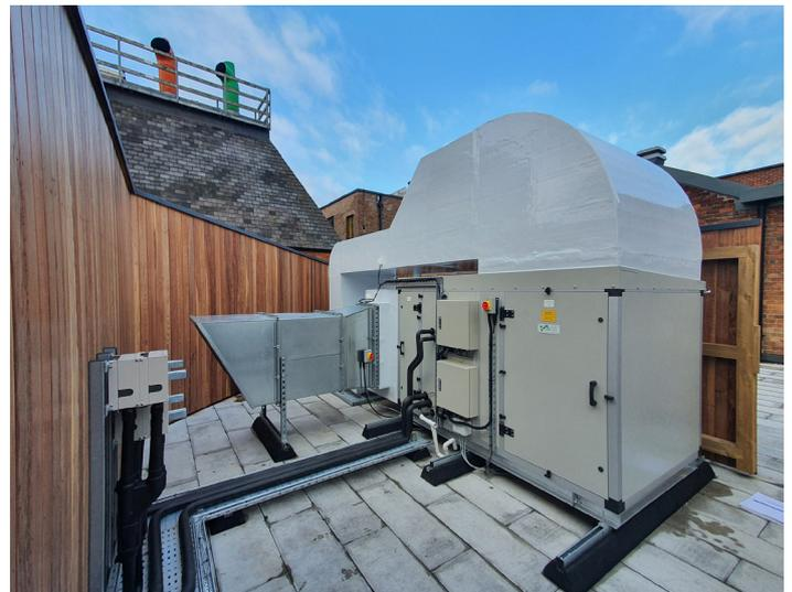
Recirculation AHU with full fresh air capabilities and direct expansion heat exchangers
