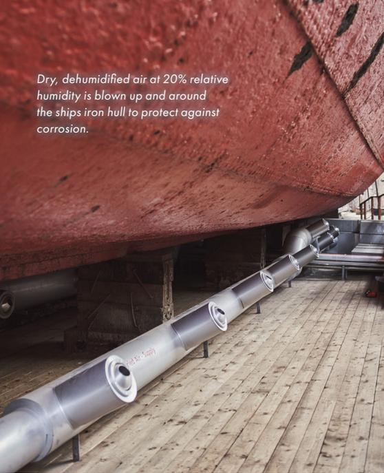
Dry, dehumidified air at 20% relative humidity is blown up and around the ships iron hull to protect against corrosion.
