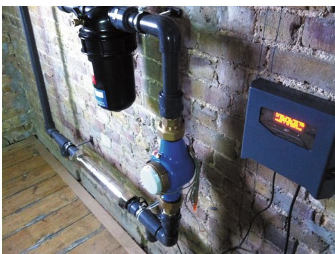
Fig D2.5 Electrolytic Scale Control Equipment showing range of 'inline anode units'
