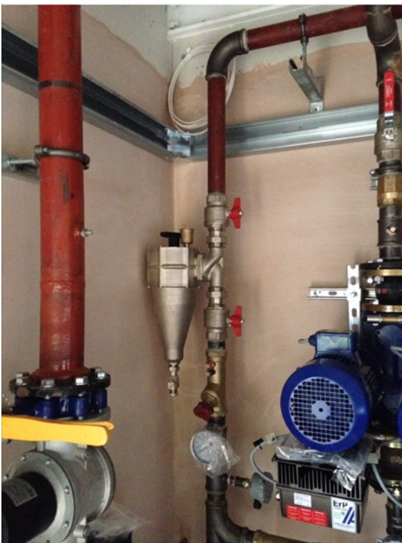
Figure A6.3.4: Hydro-cyclone Dirt Separator (1)
