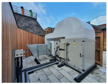
Recirculation AHU with full fresh air capabilities and direct expansion heat exchangers
