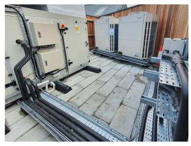
Fujitsu Airstage V-III providing direct expansion cooling and heating via AHU
