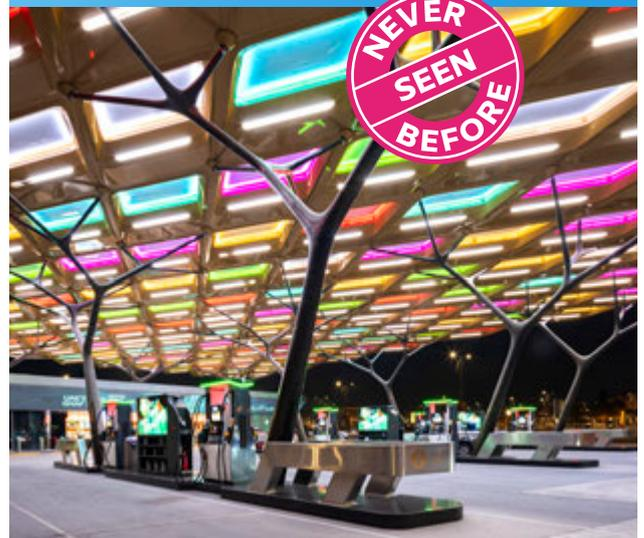
The UAE's national tree is renowned for its resilience to harsh weather conditions. The Service Station of the Future is built on an exoskeleton based on the ghaf tree structure, supporting a cutting-edge, solar-powered, carbon-fibre canopy.
